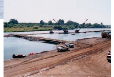
In-river construction using longitudinal berm
