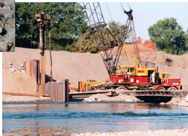
Installation of one of the sheet pile cutoff walls
