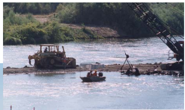
In-river construction using drag line
