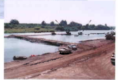
In-river construction using longitudinal berm
