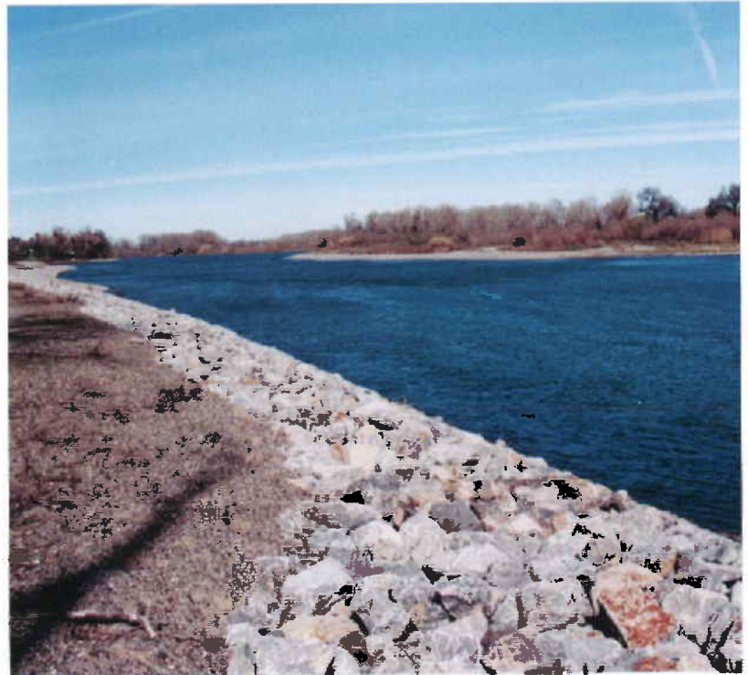
Upstream view of Sacramento River gradient facility and rock slope protection
